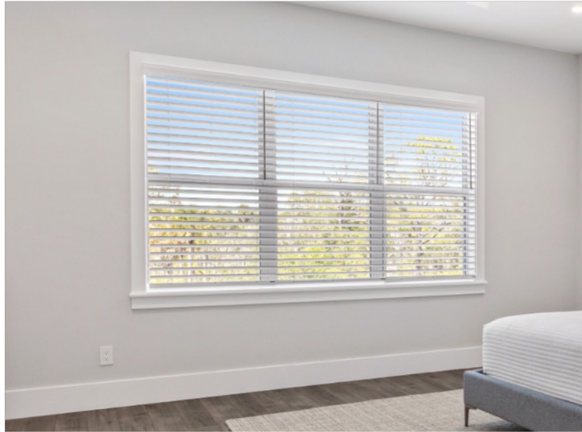
8 INCH FLAT BASEBOARDS & WRAPPED WINDOWS & SILLS
